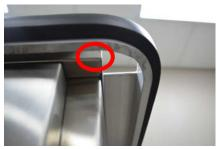
Reinforce top corners with TIG weld instead of spot weld
